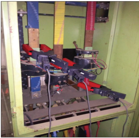
Figure 1: Medium voltage panel measurement
